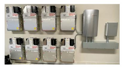
Figure 1: Backup system - IQ Battery 5P (without cover)
